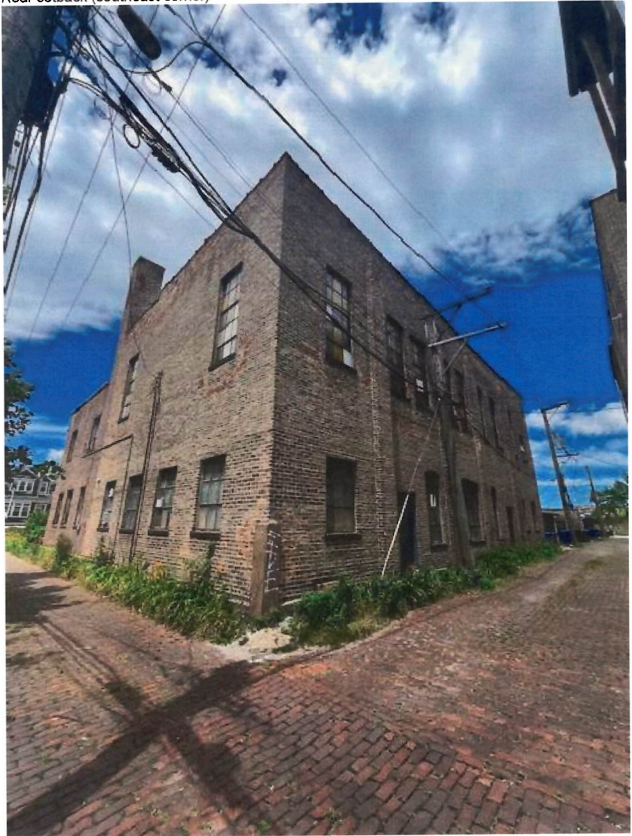
Rear setback (southeast corner)
