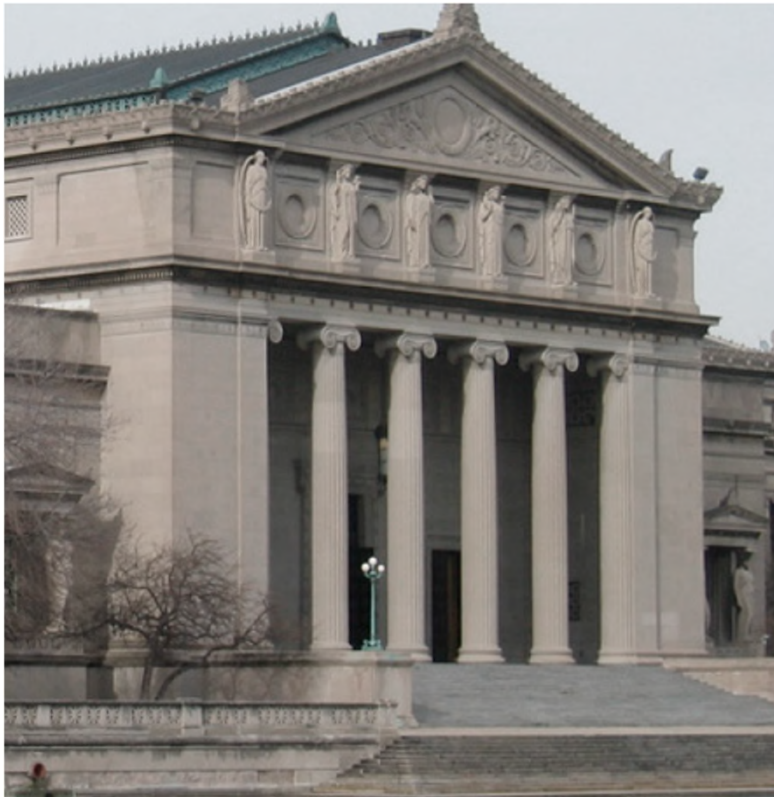
Photograph of the Existing South Portico Architect: Charles B. Atwood for D. H. Burnham & Co. Circa 1929-40
