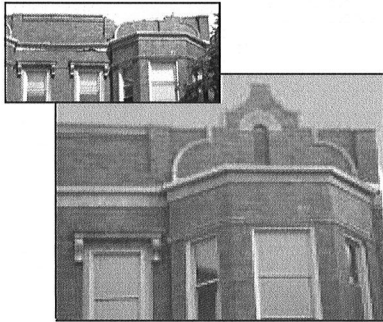
The crumbling facade on this apartment building at 4343 S. Michigan Avenue was restored to its original state through the Troubled Buildings Initiative.
