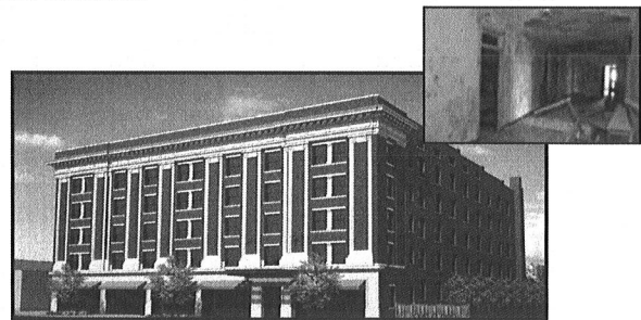
The vacant, Classical Revival-styled Strand Hotel will house 63 studio and one-bedroom apartments following a $23 million, mixed-use redevelopment.
