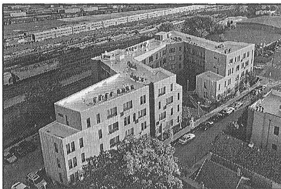
The construction of Casa Queretaro at 1614 S. Damen in the 25th Ward replaced abandoned silos on a City-owned brownfield site with an award-winning four-story building containing 45 units of affordable rental housing.
